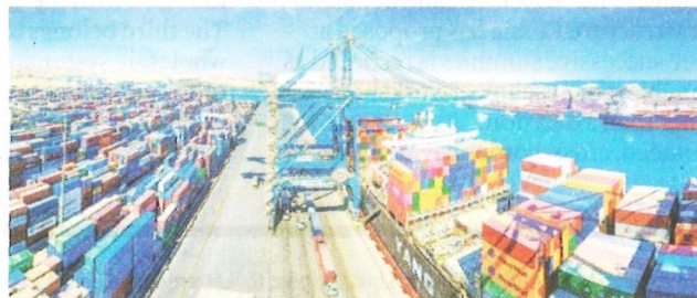
STRUCTURAL SHIFT. DP World's Sokhna terminal in Egypt handles feeders ranging from 1,200 TEUs to 5,000 TEUs
