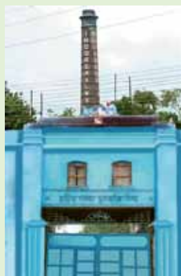
Indore Malwa United Mills (once owned by Govindram Seksaria, now taken over by National Textile Corporation)
